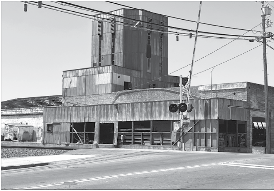
The building at the corner of Magnolia and Virginia Streets has become of concern to neighbors living in the area. Photo by Lisa Mankins
