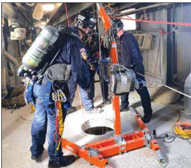
Here you can see CALFIRE technical rescue team members setting up a rope system as they prepare to enter a small circular entrance to the silo located on the floor. The large orange apparatus seen in the center of the photo is Sun West Millings equipment used to raise and lower their workers into the silos, which was suspected to have malfunctioned. Photo provided by CALFIRE/ Butte County
