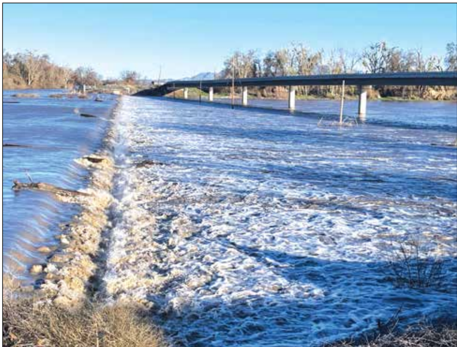
As designed, the Sacramento River began overflowing the Tisdale Weir again (January 10, 2023), with water flowing into the Sutter Bypass system. Photo courtesy Sutter County
