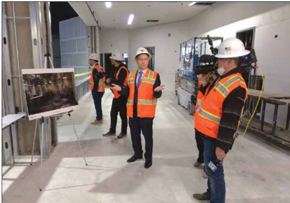
Mark Birtha, President of Hard Rock Hotel & Casino Sacramento at Fire Mountain, shares the view from the mezzanine level just above the VIP skybox. Photo by Paul Scholl
