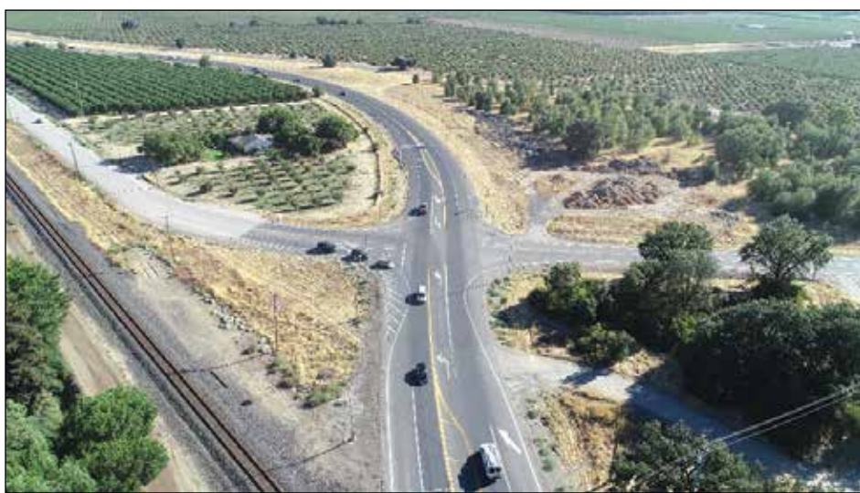
Roadway changes include no left turns to Live Oak Blvd., at Encinal Road on State Highway 99. Photo: Caltrans
