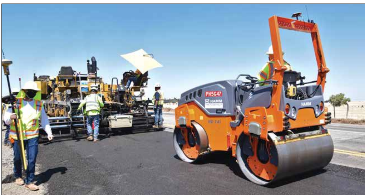
The Butte 162 pilot project is the first state highway section to use 100 percent recycled material. Photo: Caltrans
