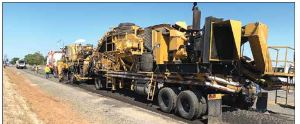
A recycling train of equipment will grind up the top 3 inches of Butte 162 pavement and then mix the grindings with a liquid plastic polymer binder. Photo: Caltrans
