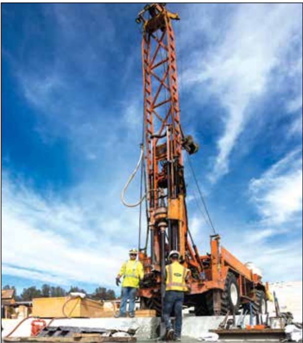
A crew from Sacramento Drilling Inc. drills a vertical drain into the Lake Oroville emergency spillway splash pad to release groundwater from beneath the splash pad at the Butte County, California site. Photo by Ken James/California Department of Water Resources
