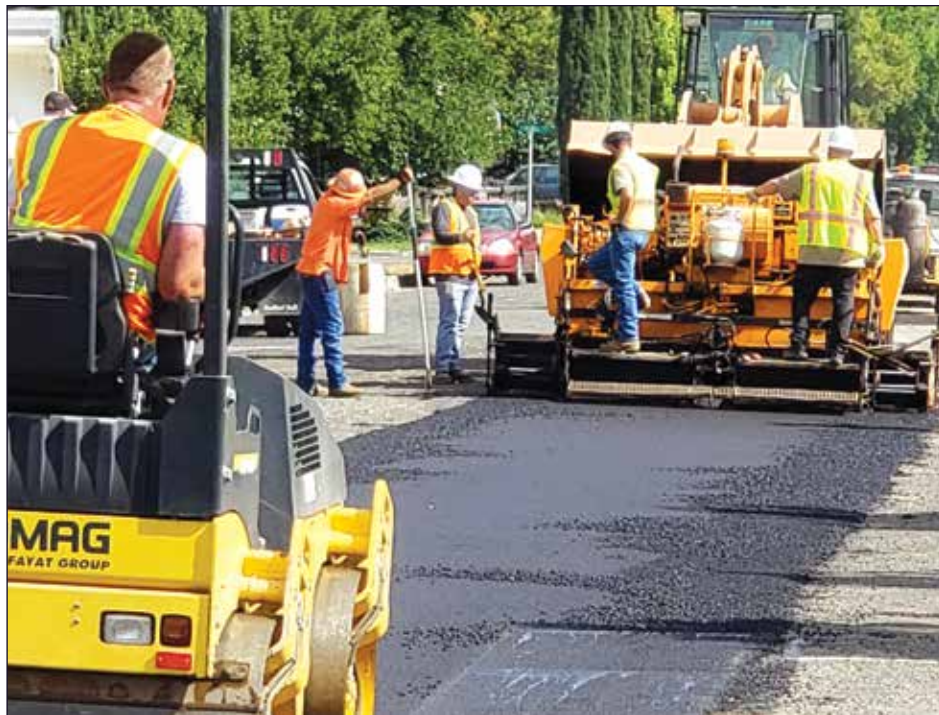
Gridley City crews hard at work laying asphalt and repaving a section of a Gridley street. Photo provided by Daryl Dye
