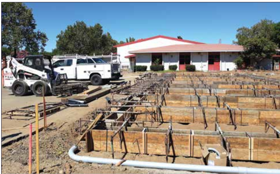
The foundation infrastructure of the old portables located between the library and cafeteria at Sycamore are exposed, allowing crews to plumb the new classrooms for water and address drainage issues that have plagued the school. Photo by Seti Long
