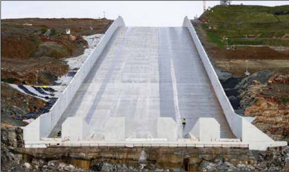
The reconstructed Oroville Dam spillway. Photo courtesy DWR
