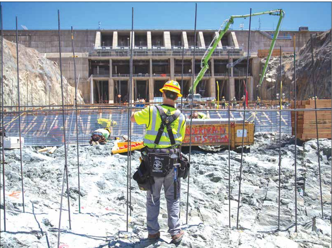
A worker from Kiewit Infrastructure uses rebar to construct a stay-form that will hold leveling concrete in place on the upper chute of the Lake Oroville main spillway in Butte County, California. Photo taken July 5, 2018. Photo by Ken James, California Department of Water Resources
