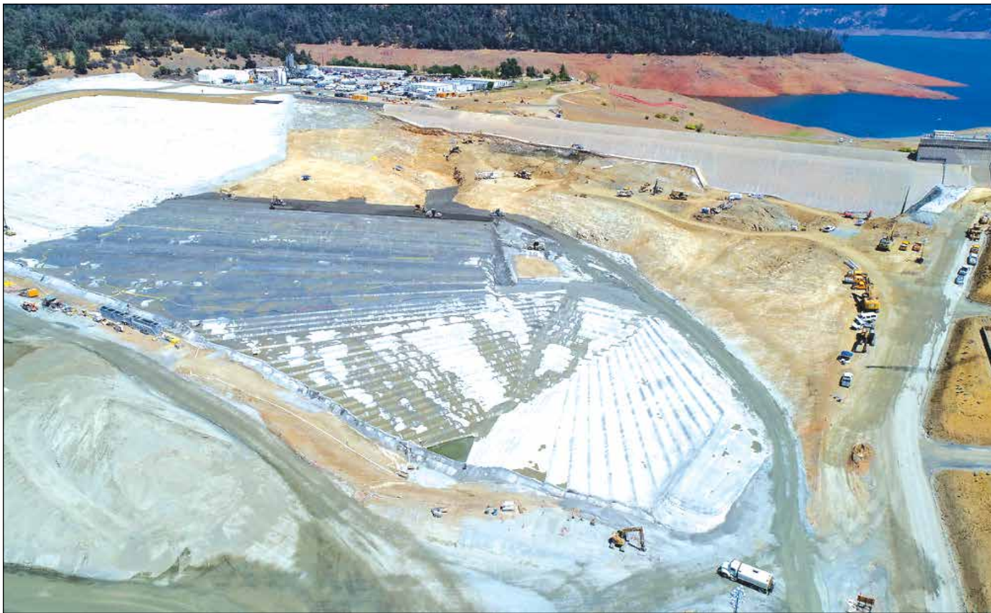
A drone provides a bird's-eye view of the Lake Oroville emergency spillway and the second phase of construction of the roller-compacted concrete splashpad on the hillside above the secant pile wall at the Butte County, California site. Photo taken August 15, 2018. Photo by Ken James, California Department of Water Resources
