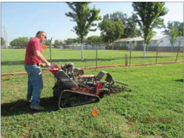
TRENCHING WORK was the first step. Steve Williams, of Max's Miracle Ranch, began the project by digging trenches with a trencher donated by Rental Guys.
