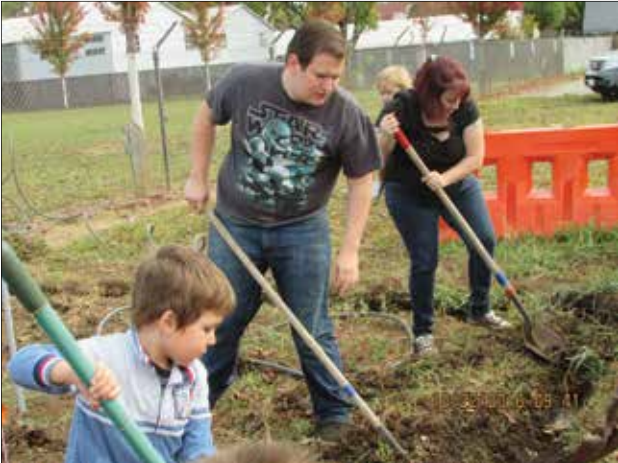
DIGGING BY HAND Volunteers helped widen trenches when a larger cement foundation was required for the brick. L to R AJ Roberts, Jack Winters, Amaya Clower, Kristey Clower
