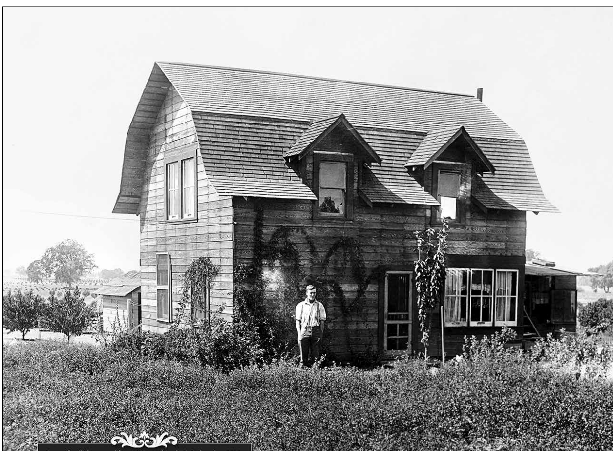
The Graves' barn served as the family home for many years. Photo courtesy Doris Graves Chez.
