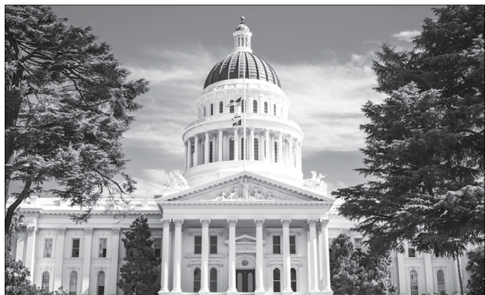
Substantive changes were made to the Capitol Annex Project's Environmental Impact Report (EIR), resulting in violations to the California Environmental Quality Act (CEQA). MPG file photo
