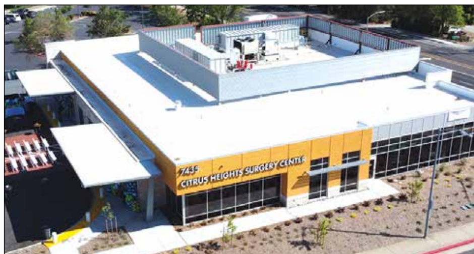
The $13 million finished project is a 16,000 square-foot ambulatory surgery center in Citrus Heights, located at 7435 Stock Ranch Road, on the corner of Stock Ranch and Sylvan roads in Citrus Heights. Photo courtesy of Dignity Health
