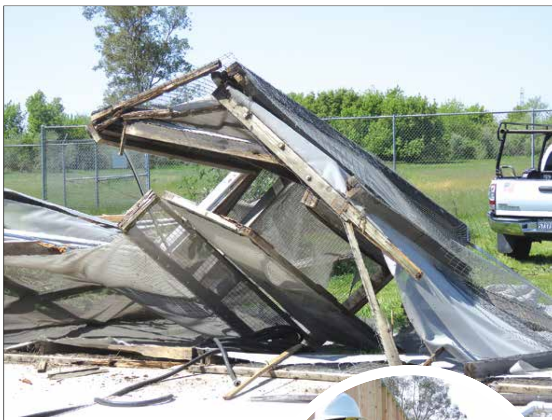
Above: February's gusty winds did some serious damage. Right: Volunteer workers employed by Wells Construction Corporation erect new walls for the Sacramento Wildlife Care Association's new aviary.
