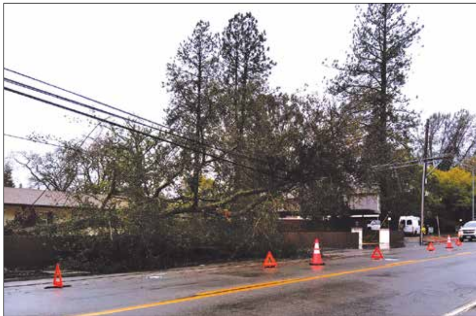
Storms knocked out electric power lines around the county such as this one on Sutter and Olive Lane, Carmichael, CA. Photo by Patrick Larenas
