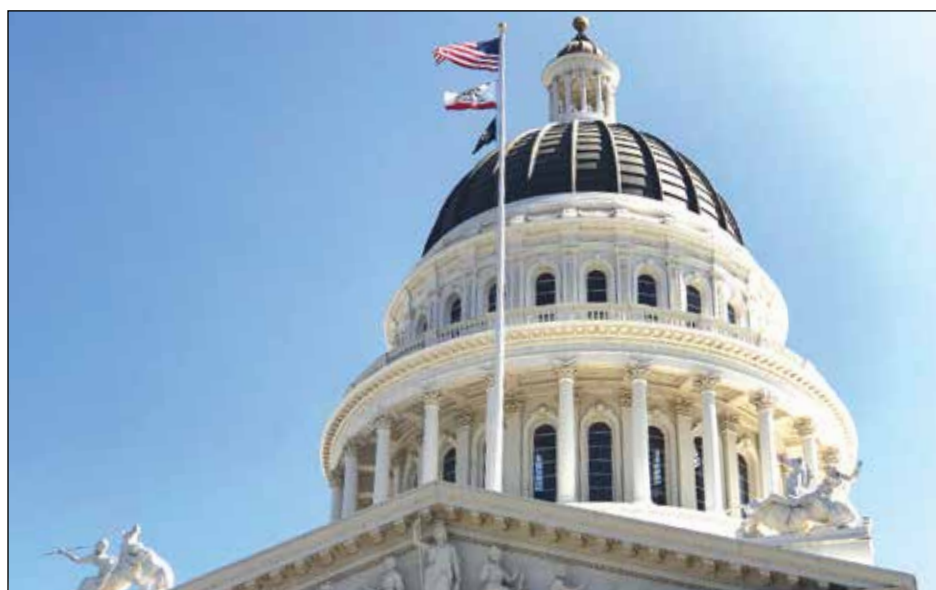
The design plans for the Capitol Annex Project aim to highlight views of the iconic dome of the State Capitol's historic west wing. Photo provided by Assemblyman Ken Cooley
