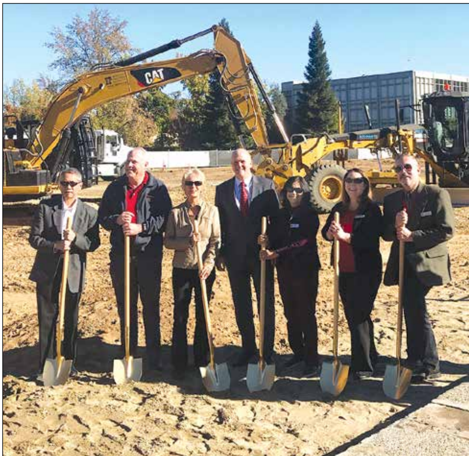
The STEM groundbreaking kicks off the next phase. ARC has launched a major fundraising effort for STEM Innovation and 21st Century Science. Photo by Tatyana Torgashev, courtesy ARC
