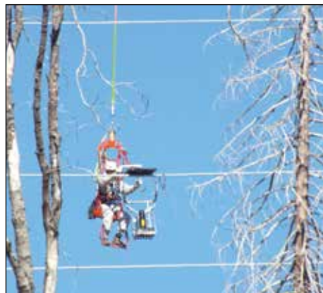
Suspended from a helicopter, a lineworker conducts X-ray photography on a SMUD transmission line in the Sierra. The work helps SMUD identify potential issues in advance so they can be repaired and help avoid power outages that could affect thousands of customers. Photo courtesy SMUD
