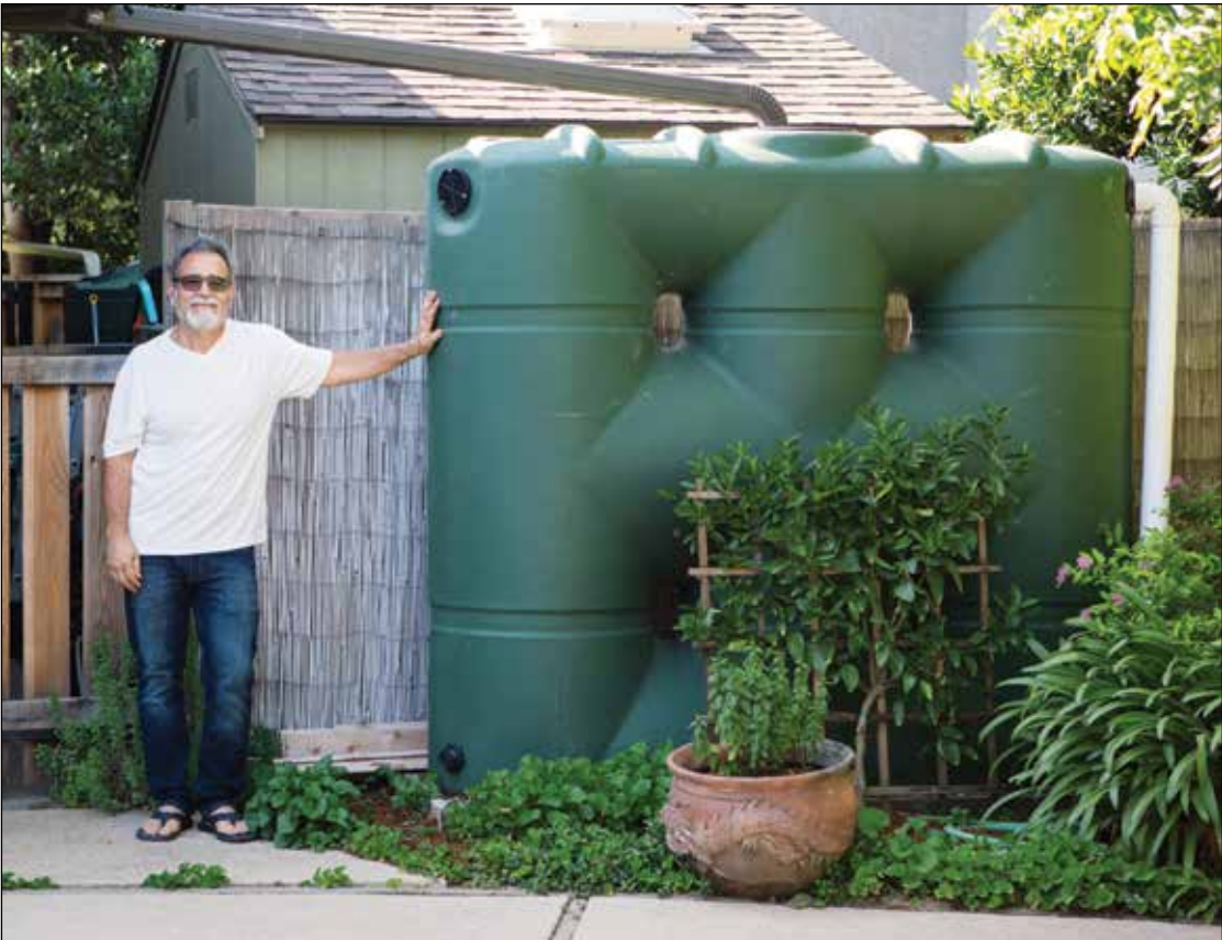
Their new gutters feed into five cisterns, three 860 gallon tanks and two 530 gallon ones, that will help to provide water for their landscape.
