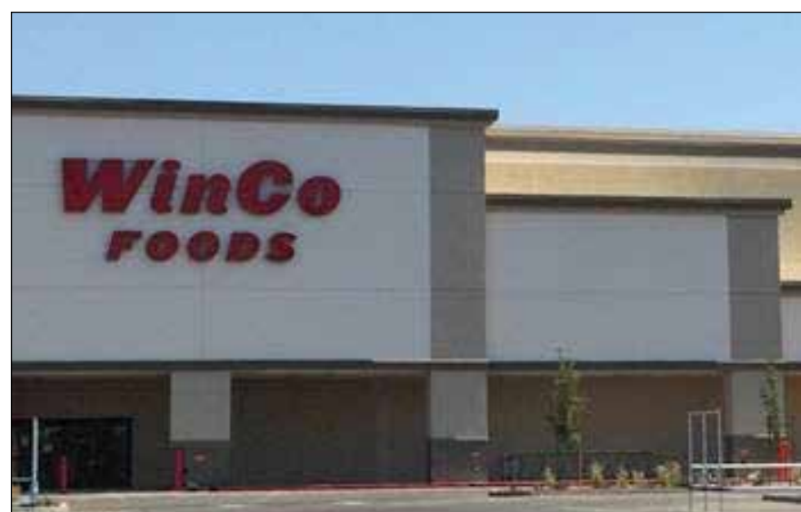
the new WinCo Foods building is approximately 100,000 square feet and will be open 24 hours a day, seven days a week.
