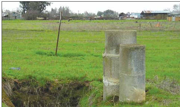
Children, animals, and even adults can fall into abandoned wells causing injury or death. Open pit wells and large-diameter drilled wells are particularly hazardous and often are hundreds of feet deep. Photo courtesy of Sacramento County.
