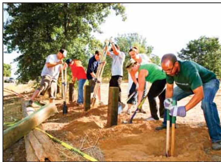
A Saturday working bee at Jan Park benefited by the efforts of over 150 volunteers. Work teams sank bollards around the reserve perimeter to prevent unlawful vehicle access. Photo by Susan Maxwell Skinner.
