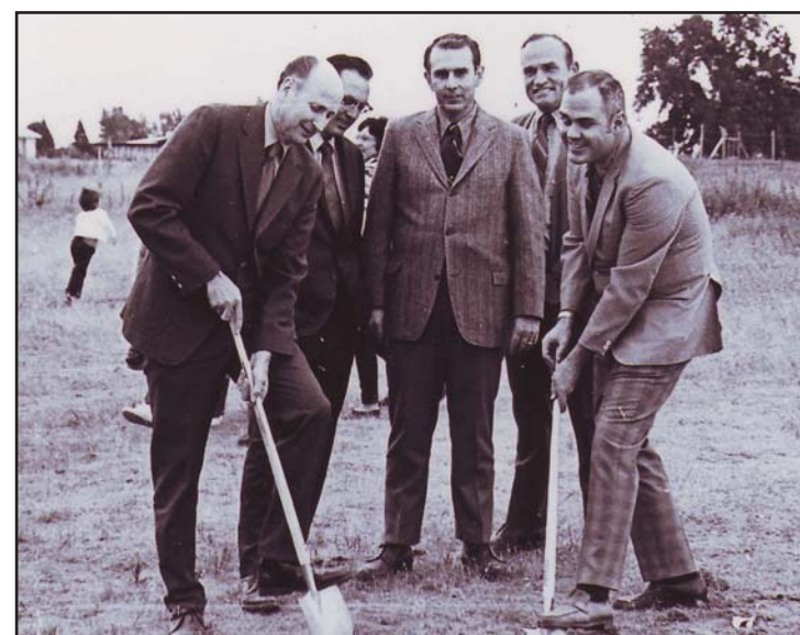
Groundbreaking for a new Stake Center
