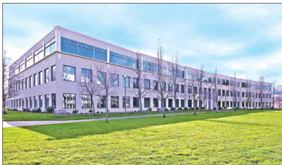
One of California's largest semiconductor projects will move into White Rock Corporate Campus, creating up to $1.2 billion in annual economic impact for the capital region. Photo courtesy of the City of Rancho Cordova
