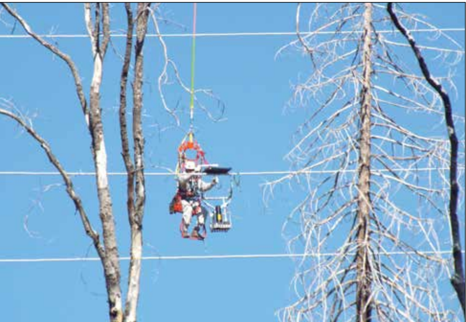
Suspended from a helicopter, a lineworker conducts X-ray photography on a SMUD transmission line in the Sierra. The work helps SMUD identify potential issues in advance so they can be repaired and help avoid power outages that could affect thousands of customers. Photo courtesy SMUD
