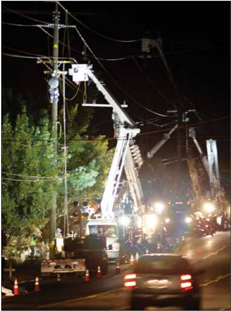
SMUD line crews replaced power poles on Hazel Avenue overnight June 28/29. The poles support 69,000-volt power lines that are the backbone of the SMUD system that delivers electricity to homes and businesses. The work is part of SMUD's efforts to enhance the SMUD grid's reliability.
