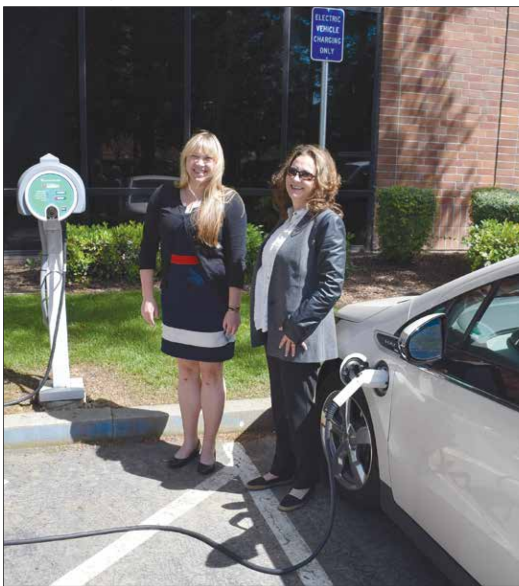
Rancho Cordova City Hall employees utilize the 240-volt charging stations for hybrid and electric cars. Photo by Ashley Stidham
