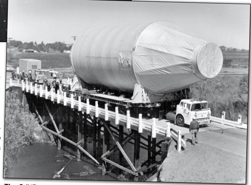
The S-IVB stages travelled from the Bay Area up the Sacramento River on barges. Once they arrived at the specially built dock in Hood, they were transferred to flatbed trailers for the trip to the test site traveling at seven miles per hour on narrow county roadways and bridges. Workmen along the journey had to lift telephone wires and trim trees to enable the stage to make the journey to the test center. Photo courtesy of Center for Sacramento History, Douglas Aircraft Company/NASA Employee Collection, 2014/015.
