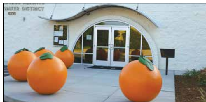
Even the oranges have a story at the newly refurbished Citrus Heights Water District's Administration Offices. The oranges are made of concrete and were purchased from a firm in San Jose. The leaves were crafted by staff from the remains of old shovels. Photo by Elise Spleiss
