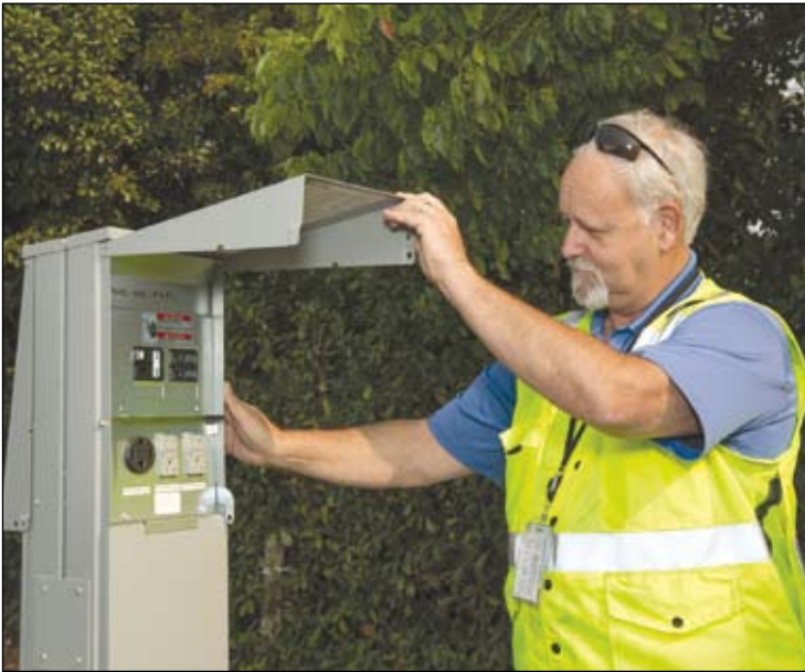
Sacramento Municipal Utility District (SMUD) Program Manager David Hatfield inspects newly installed “shore power” electric hookups at the Sacramento 49er Travel Plaza, a truck stop near the interchange of Interstates 80 and 5. By providing utility power where big-rig drivers spend their rest periods, truckers can plug in their rigs to electrical outlets and avoid idling their engines. By doing so, truckers save money and harmful emissions are reduced.
