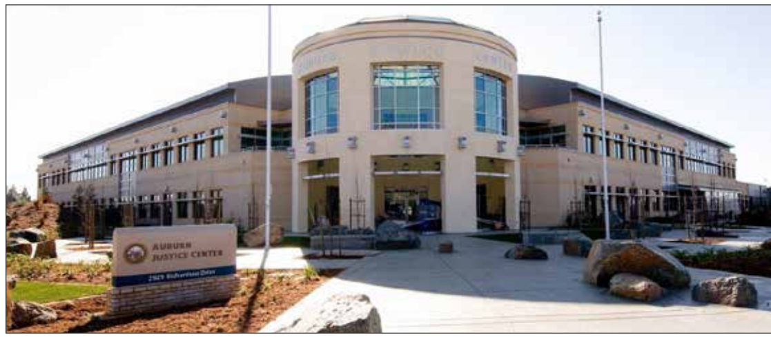
Auburn Justice Center. Photo courtesy Placer County
