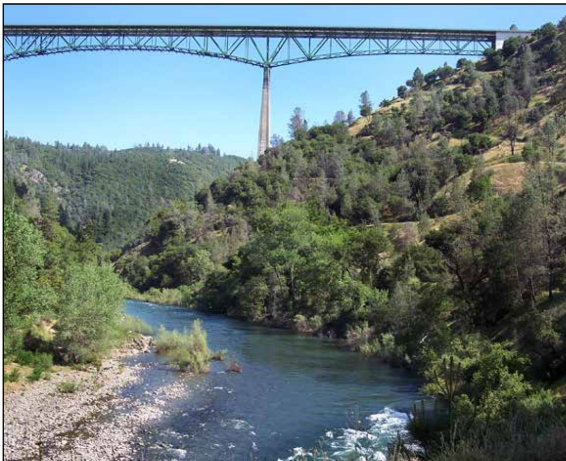
The spectacular view of the Foresthill Road Bridge on the way to Lake Clementine.
