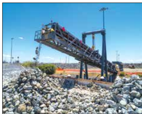
Rock is loaded onto barges at the California Department of Water Resources Weber Rock Yard near the Port of Stockton, California. The purpose of the rock barrier is to prevent the Delta from becoming too salty for irrigation, drinking water, or fish. Photo by Florence Low/California Department of Water Resources
