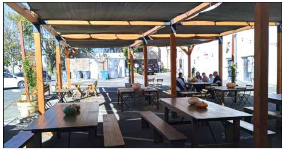
This spacious pergola was built and utilized in Ferguson Alley by the restaurant owners who have a backside to it: Rosemary's Farm to Fork, Dawson's Bar and Grill, and Bangkok Garden. But, it cannot even be utilized for outdoor dining for the next three weeks of the Deep Purple pandemic restrictions. All restaurants under this order allow take out and pick up only. The Solano Small Business Development Center is offering programs that can help small business owners stay in business. Meanwhile, please order out to support our Dixon merchants. Photo by Debra Dingman
