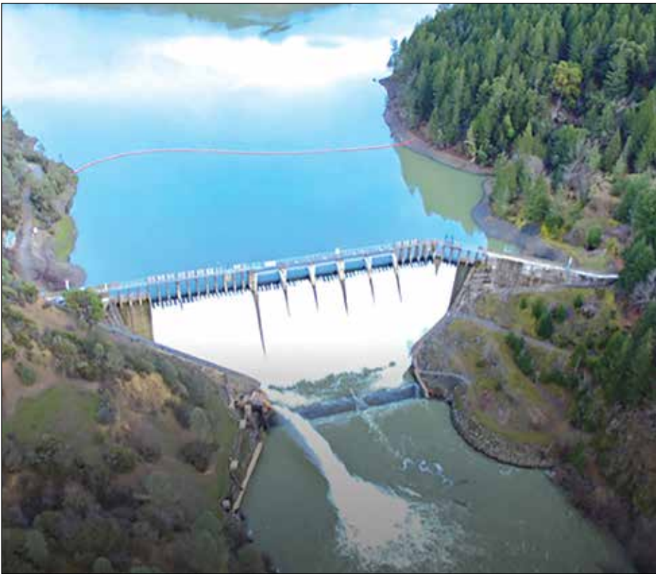
The Scott Dam on the main stem of the Eel river holds water for the Lake Pillsbury reservoir.
