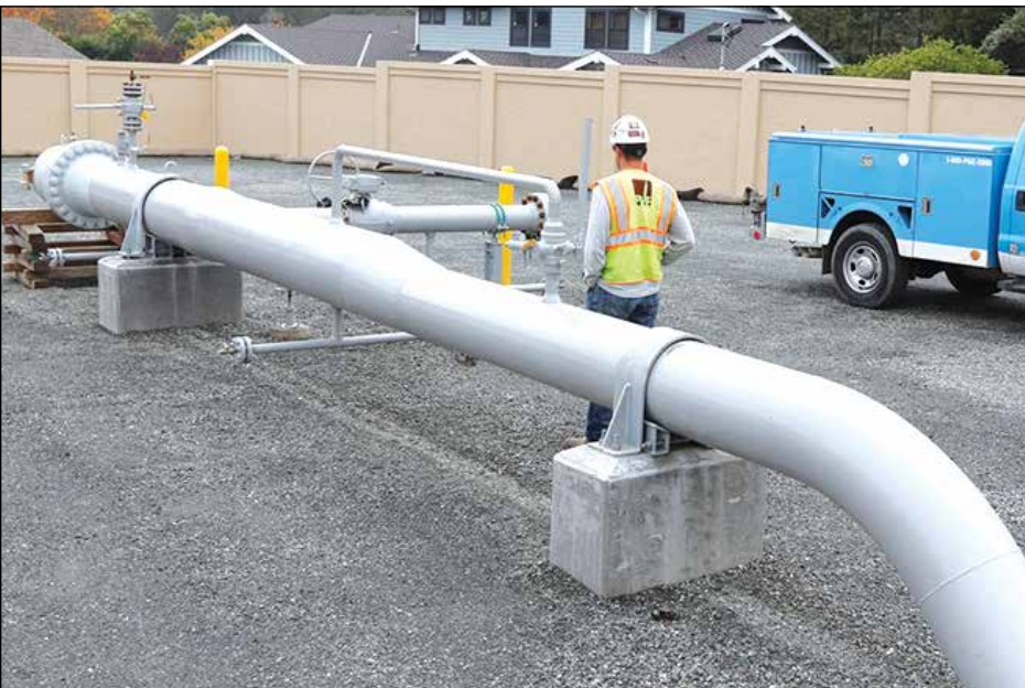
A PG&E gas robotic pig launcher/receiver site in Contra Costa County. Technology gives detailed look inside natural gas pipelines to confirm safe operations. Photo courtesy of PG&E
