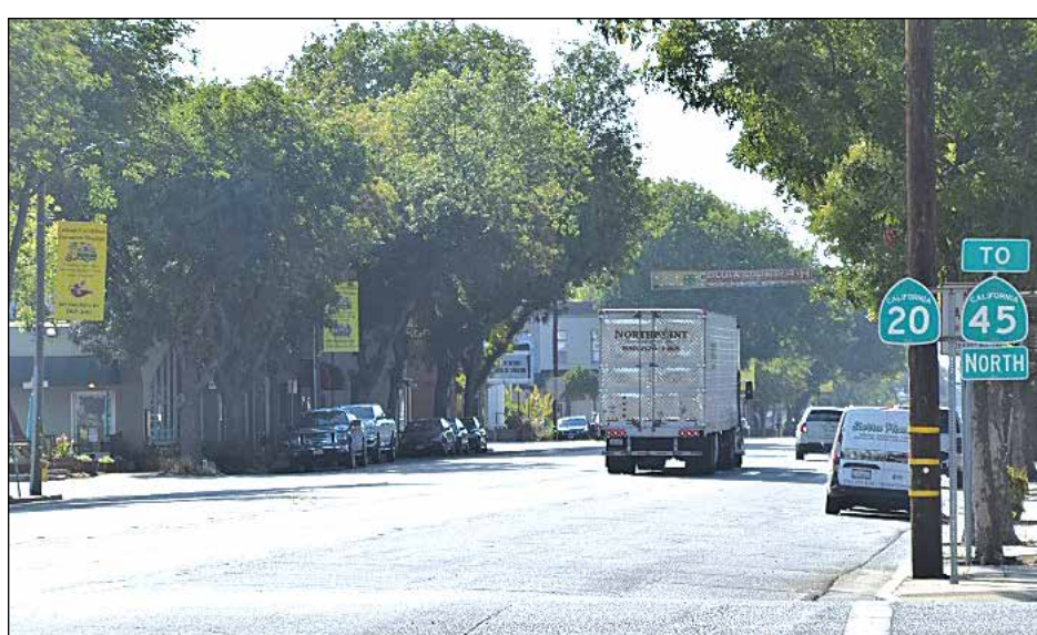
The main thoroughfare through Colusa is undergoing roadwork through the month of October. Photo courtesy of Caltrans
