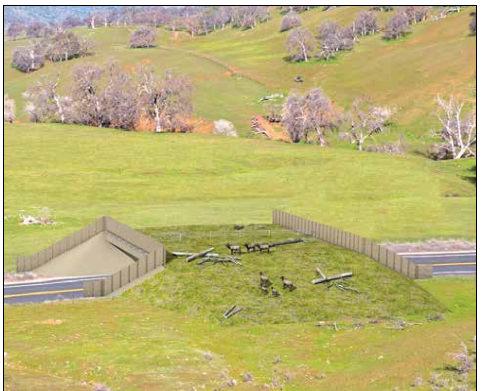
The proposed wildlife overcrossing on State Highway 20 in Colusa County. Photo courtesy of Caltrans
