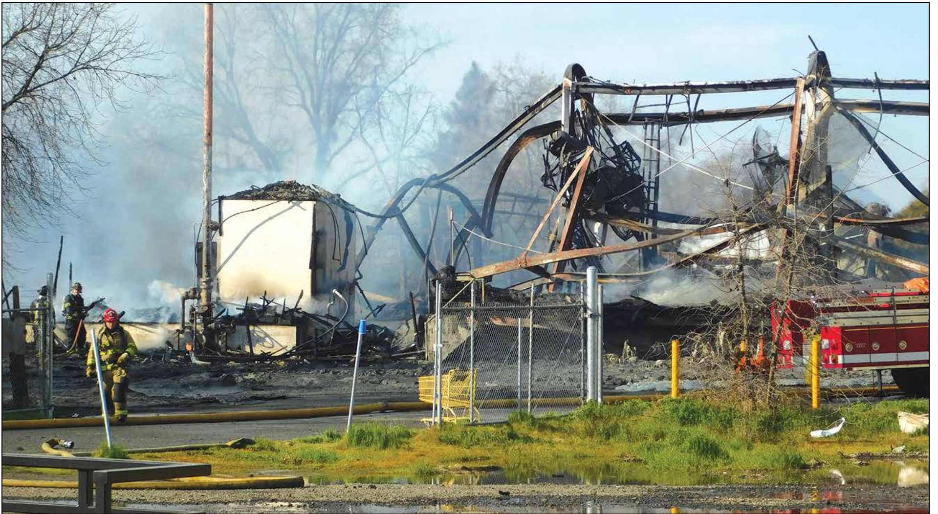
The Diamond Walnut Factory in Live Oak was quickly reduced to rubble as a blazing fire tore through the structure early Friday morning. Photo by Seti Long
