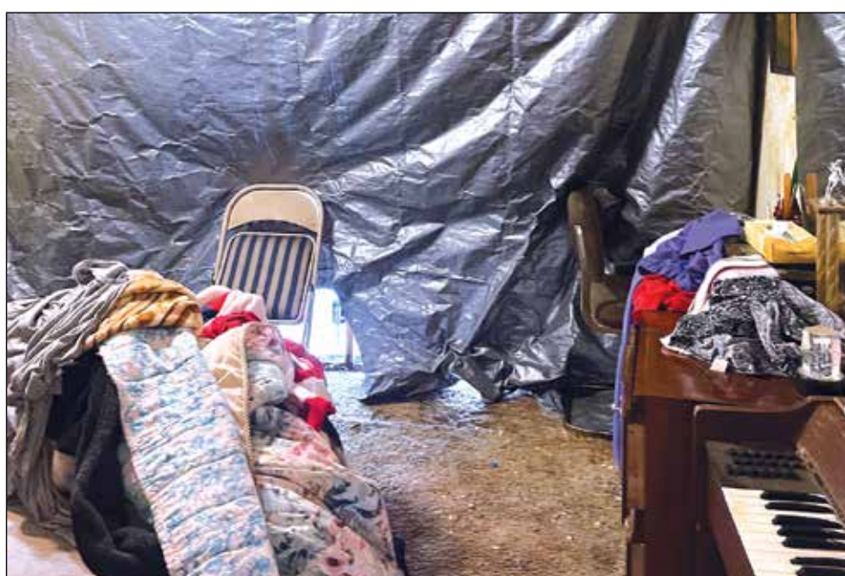
An effort was made by the resident to shield the interior from the outside damp elements. Photo: EXP Realty of California
