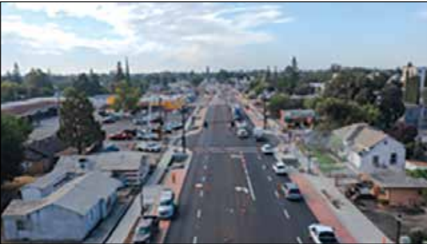
Highway 99 near Kola Avenue in Live Oak has been widened from two to four lanes with left turn lane access. Improvements also include sidewalks and lighting enhancements, improving mobility for all. Photo courtesy CalTrans
