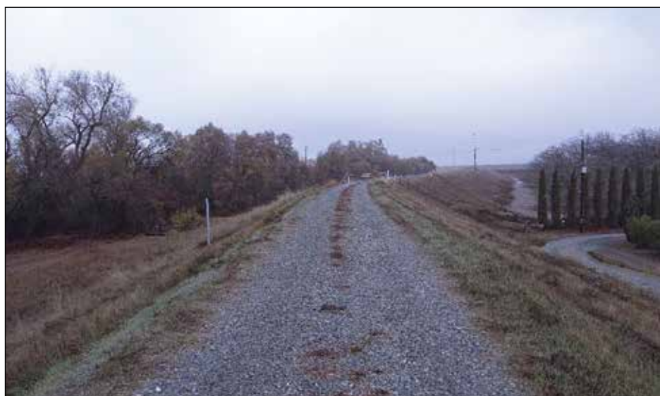
The toe access corridor project site in Reclamation District 10, north of Marysville. Photo courtesy Yuba Water.
