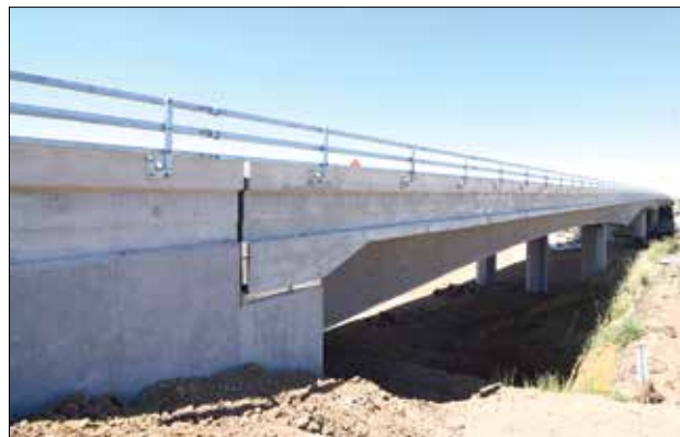
New Simerly Slough Bridge Made Possible by SB 1. Photo courtesy CalTrans
