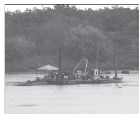
Hydraulic Dredge Yuba/Feather River
