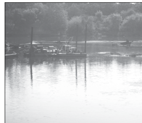
Hydraulic Dredge at Yuba City.
