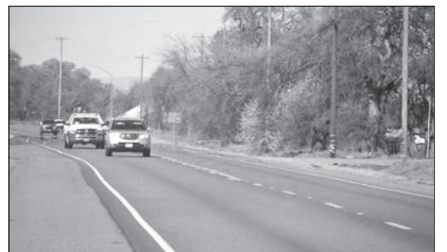
It took a lot of hard work by our partners and Caltrans to get this stage. We’re excited to begin construction on this segment. Photo courtesy CalTrans
