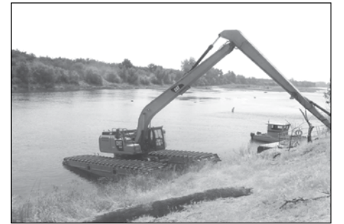
Track Layer Dredger
