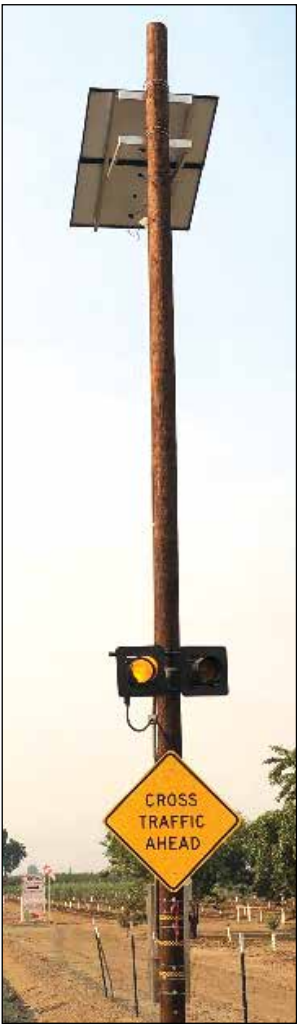
Solar-powered roadside amber beacons flashing systems have been placed at two intersections on state highway 70 north of Marysville. Photo: Caltrans
