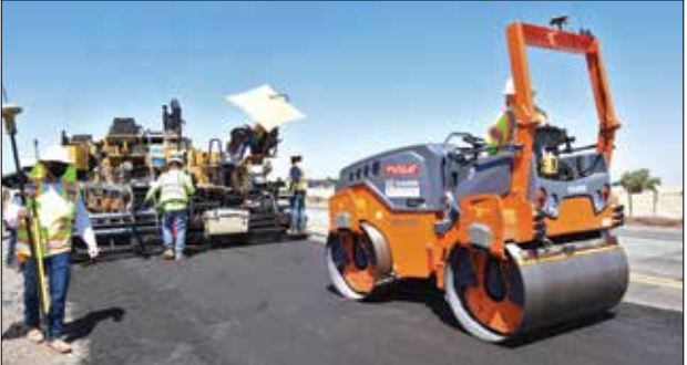
The Butte 162 pilot project is the first state highway section to use 100 percent recycled material. Photo: Caltrans
