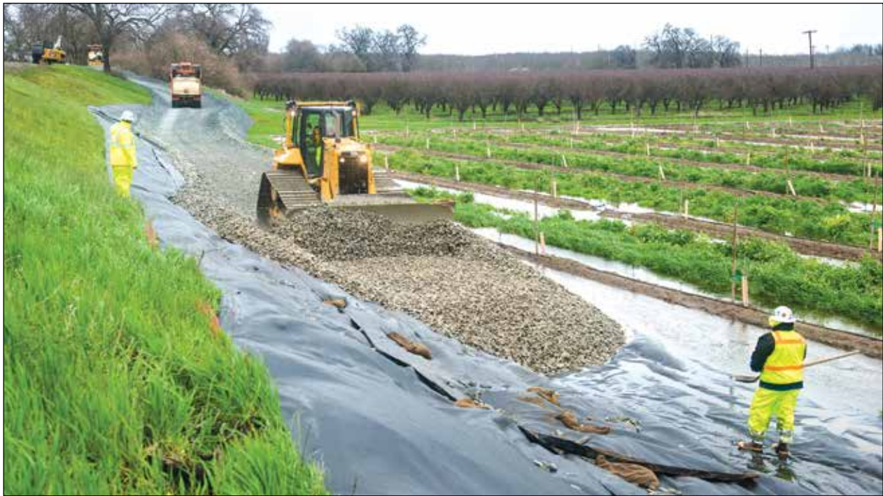
Levee work done on the east bank of the Garden Highway in Nicolaus, California. A stability berm is constructed to support the levee at the damaged location, February 17, 2017. The site is approximately 1 mile north of the Feather River and Sacramento River confluence in Sutter County. Photo: Florence Low / California Department of Water Resources
