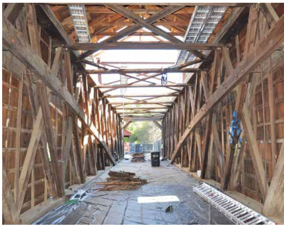
Photo taken from inside facing south by Marc Wetherbee
